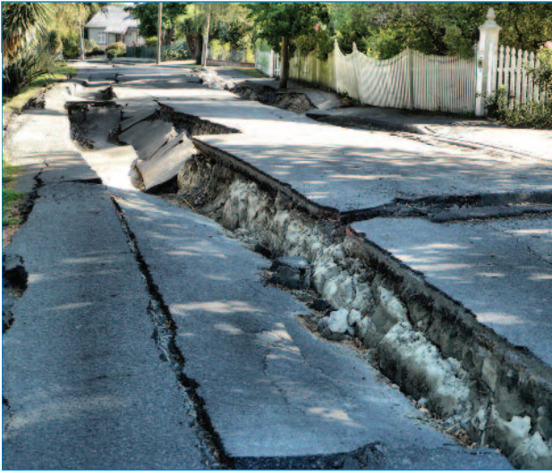
Damage to a road after the 2011 earthquake, Christchurch, New Zealand.
