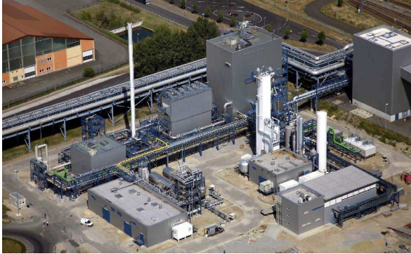
Figure 7. An oxy-combustion pilot plant capturing CO 2 from the flue gas of a coal-fired boiler in Germany. The plant size is the electrical equivalent of approximately 10 MW. (Photo courtesy of Vattenfall)
