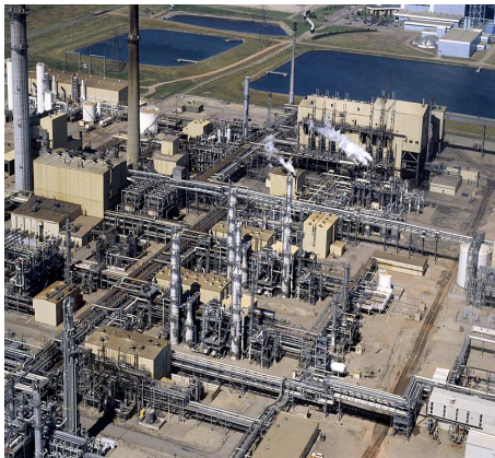
Figure 5. A pre-combustion CO 2 capture system used to produce synthetic natural gas (syngas) from coal at the Dakota Gasification Plant in North Dakota. About 3 Mt/y captured CO 2 is currently transported by pipeline to the Weyburn and Midale oil fields in Saskatchewan, Canada, where it is used for enhanced oil recovery (EOR) and sequestered in depleted oil reservoirs. (Photo courtesy of IPCC)
